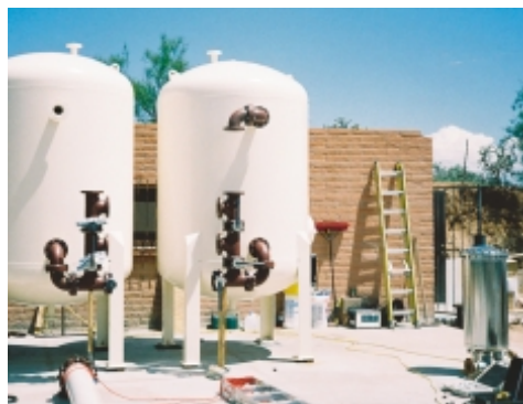
Green Valley Water Co. 1,400 gpm arsenic removal system under construction. Photo courtesy Conestoga-Rovers & Assoc.
