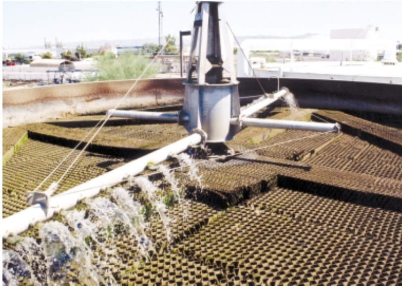
Above, Photo 7: Trickling Tanks (Photo courtesy of LES)
