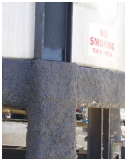
Above, right: tank stand with 2-hour fire proofing coating; above: close-up of coating
