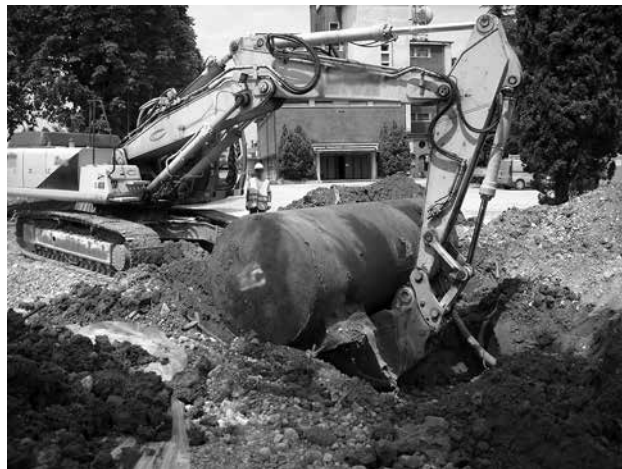
Example of UST Removal
